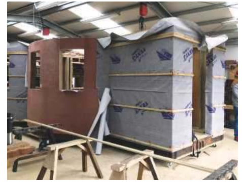
Walls being battened ready for cladding
