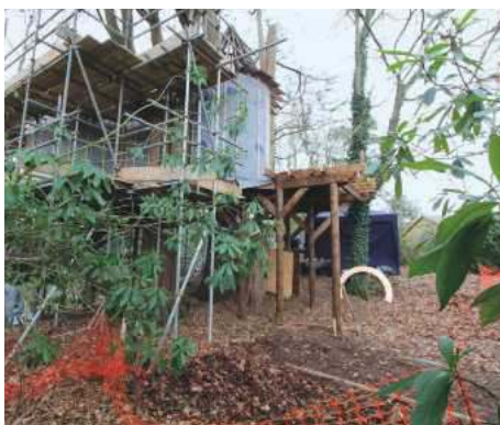
Wall batten and membrane
