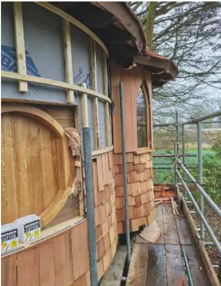
Wall cladding and fitting windows
