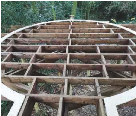
Floor joists and bottom plate
