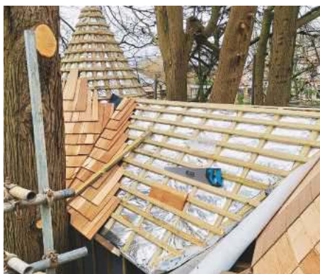
Cedar roof lining
