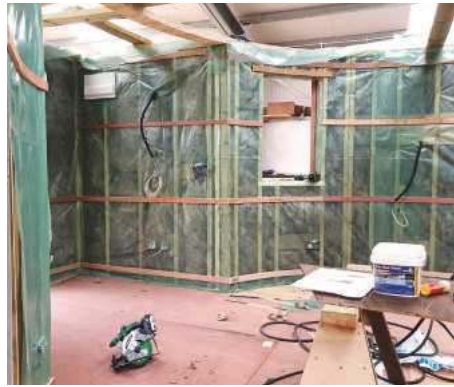
Interior walls insulated, ready for lining
