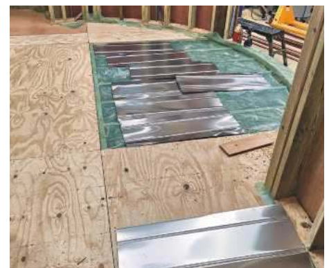
Underfloor heating trays being fitted
