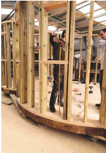
Treehouse wall framework
