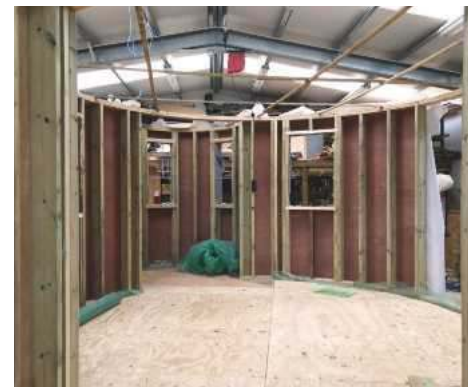
Treehouse stud walls erected
