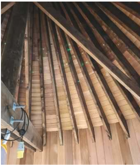
Interior cladding and second-fix electrics added
