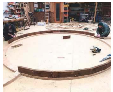
Setting out the bottom plate
