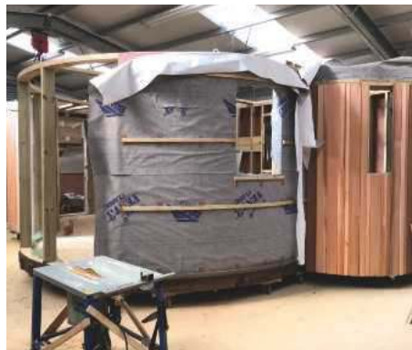
Exterior cladding being fitted...
