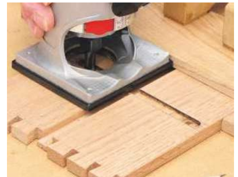
18 Cramp parts together and cut 3mm-deep housings for the dividers. Run the router against a guide batten
