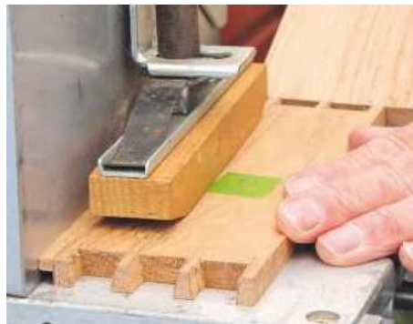
17 Create a 5mm-deep rebate along the bottom edges for the slats. Cut this on a router table to ensure accuracy
